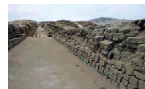
■ Calle amurallada Norte-Sur, la vía principal de Pachacámac inca, luego de trabajos de puesta en valor, vista de Norte a Sur. Foto: Krzysztof Makowski. / View of the north-south walled street after enhancement works this was the main street of Pachacámac during the Inca period. Photograph by Krzysztof Makowski.
