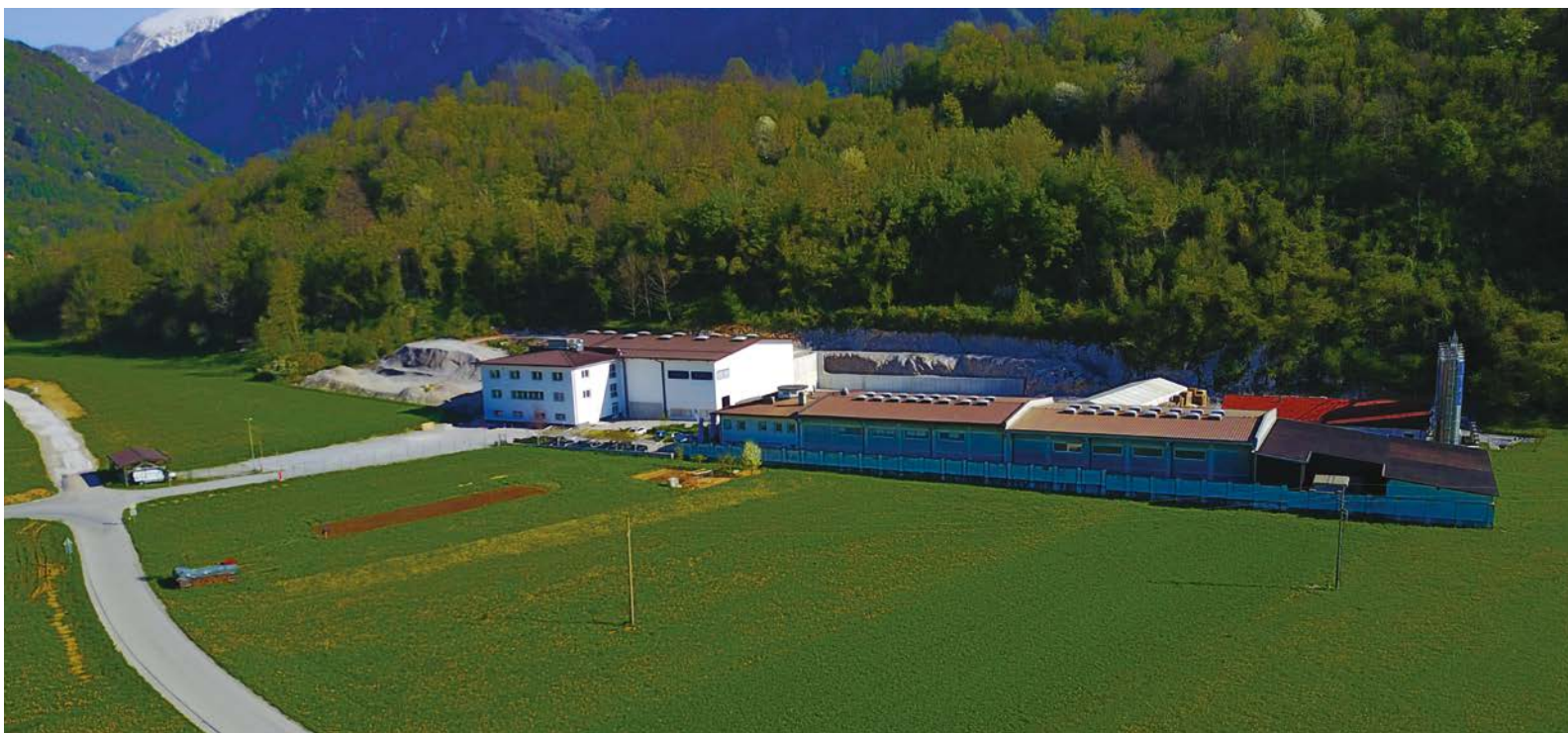
Headquarters of TERA in Volče near Tolmin
